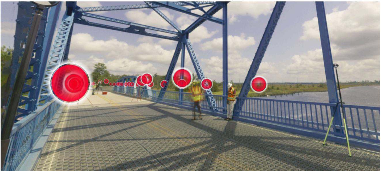
WSP field crew deploying scan targets across the bridge deck during the multi-platform reality capture survey.
