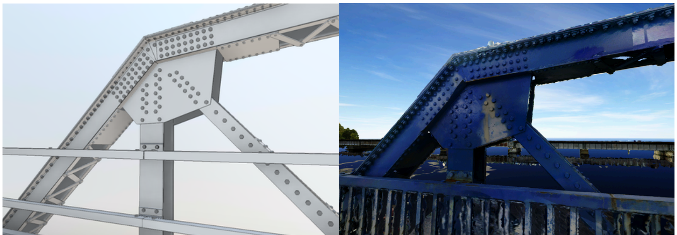
From reality capture to Revit model: the same connection, two views. Every bolt documented, every rivet modeled.
